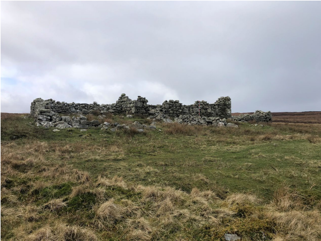
Plate 5.5: View north of the southernmost building of the Tronaster township (Asset 119)
